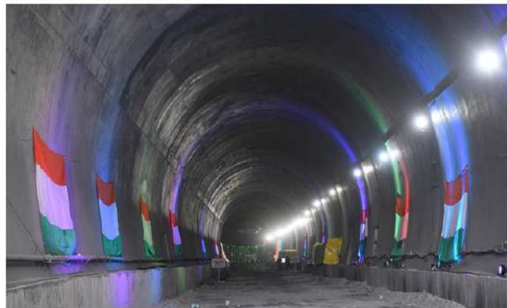
A view of the Z-Morh tunnel that connects Gagangir and Sonamarg. FILE PHOTO
